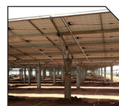
Single Post Mounts Concrete piles
