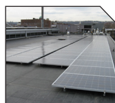
Ballasted POWER RAIL™ Mounts
