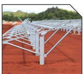
POWER PEAK Steel Structure
