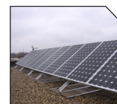
Ballasted Roof Mounts
