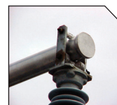
Busbar End Caps
